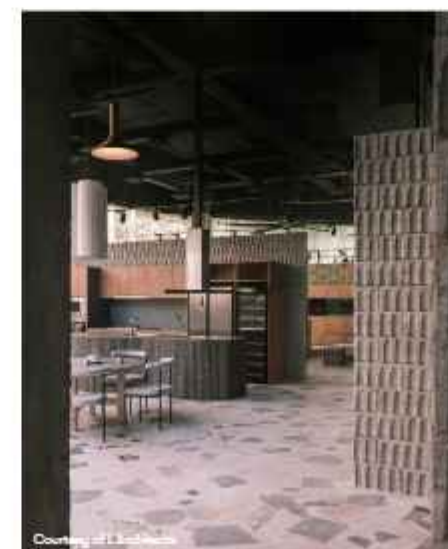
"Brick and Mortar Shop" by L Architects uses discarded "off-cut" stones and chip tiles with concrete hollow bricks to create a sensual tactile interior of material economy.
