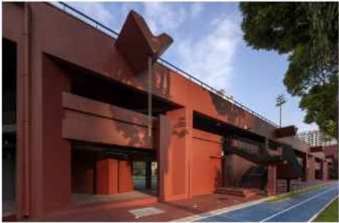
Elevated Promenade The concrete stadium seating has been re-imagined as an elevated promenade that connects the swimming complex to the indoor hall horizontally, with integrated staircases along the pathway providing vertical connectivity, 2023. (Darren Soh)
