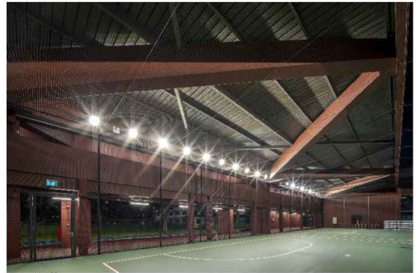
Multipurpose Court The zig-zagging cantilever beams and canopy are retained from the existing stadium architecture while the concrete tiered seating were removed to provide space for new futsal courts, surely the scene of exciting action in the evenings to come, 2023. (Darren Soh)
