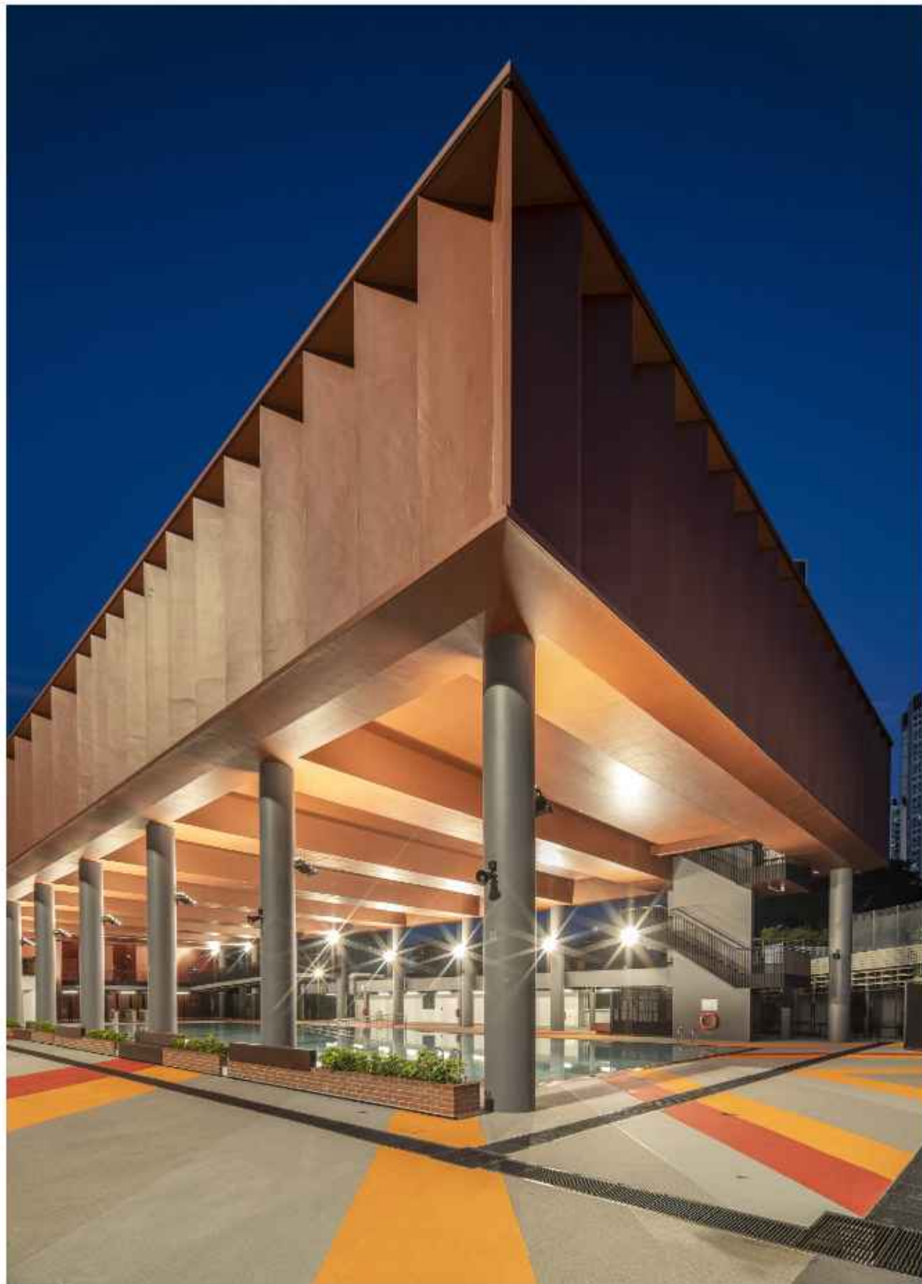
Gym Block Facade The gym block facade integrates sun-shading concrete fins against the east and west sun with glazing always facing north and south. The solitary fin touching the corner is a result of this logic, 2023. (Darren Soh)
