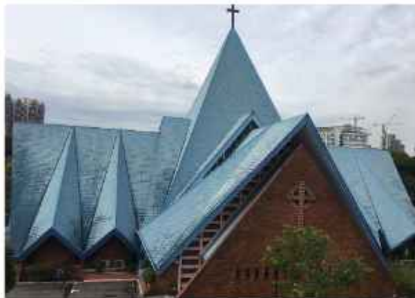
EXTERIOR VIEW: A Modern Aluminum roof replaced the original weathered blue slate tiles to provide a crisp backdrop to the religious artwork.
