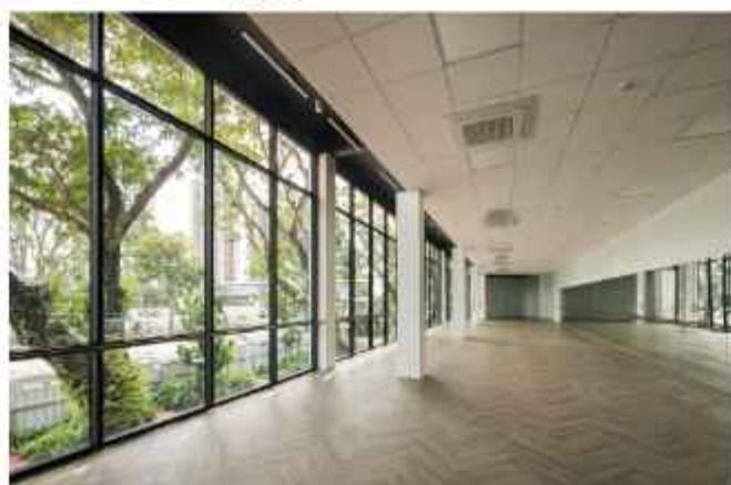
Indoor Hall The previously opaque facade was opened up with full height glazing replacing the brick infill within existing reinforced concrete frame. The former driveway and parking in front of this were also paved over to form a traffic-free connection from bus-stop to the indoor hall. Mature trees here were retained to provide shade and character. 2023. (Finbarr Fallon)
