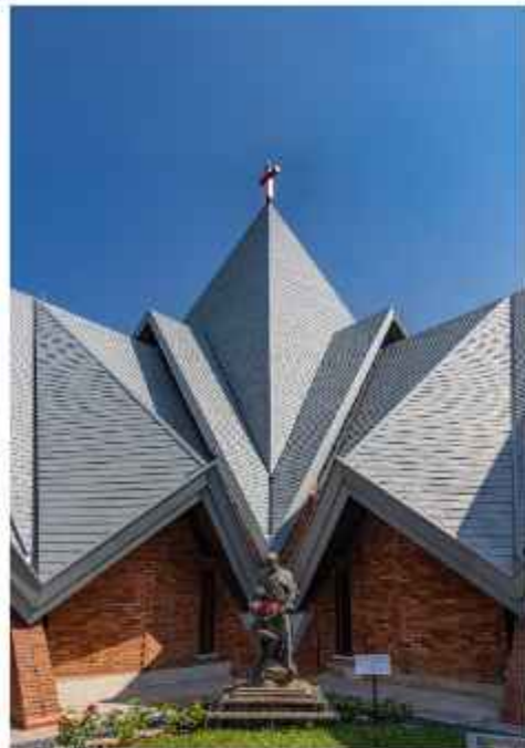
EXTERIOR VIEW: A Modern Aluminum roof replaced the original weathered blue slate tiles to provide a crisp backdrop to the religious artwork.
