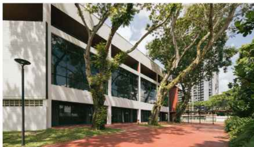
Indoor Hall The previously opaque facade was opened up with full height glazing replacing the brick infill within existing reinforced concrete frame. The former driveway and parking in front of this were also paved over to form a traffic-free connection from bus-stop to the indoor hall. Mature trees here were retained to provide shade and character. 2023. (Finbarr Fallon)
