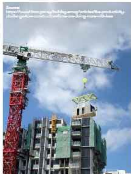
The Building & Construction Authority promotes the adoption of technology in new construction – like the use of volumetric construction (this image) and mass-engineered timber.
